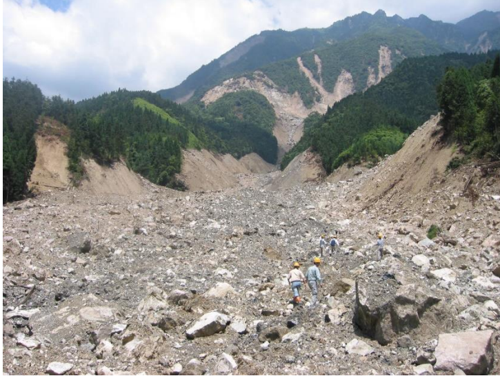
Fig. 3. Jiufengchun landslide triggered by the 2008 Sichuan earthquake, China. It started as rock fall in weathered granite (see exposed slopes in the background) and turned in catastrophic debris flow.
